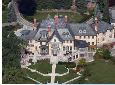
Edgemere 1502 LAKESHORE ROAD E., OAKVILLE, ONTARIO, CANADA
