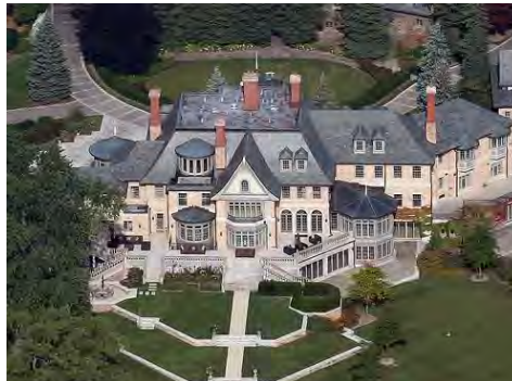
Edgemere 1502 LAKESHORE ROAD E., OAKVILLE, ONTARIO, CANADA
