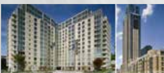
Sheepshead Residential Tower
