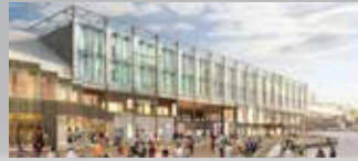
Pier 17 South Street Seaport
