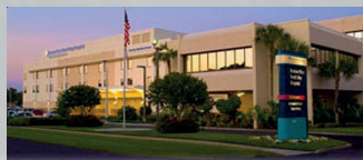
Morton Plant North Bay Hospital New Port Richey, Florida www.mortonplant.com Eng : IC Thomasson Association Incorporated
