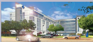
St-Joseph Women's Hospital Tampa, Florida www.sjbhealth.org Eng: Smith, Seckman, Reid Engineering
