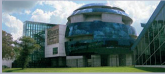
Museum of Science and Industry Tampa, Florida www.mosi.org Eng: Advance System Engineering
