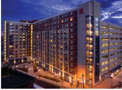
Rutgers University Apartments 604 Bartholomew Road Piscataway, NJ 08854
