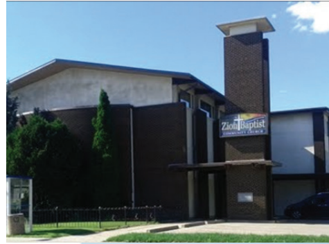
Zion Baptist Church 9802 76 Ave NW, Edmonton, AB
