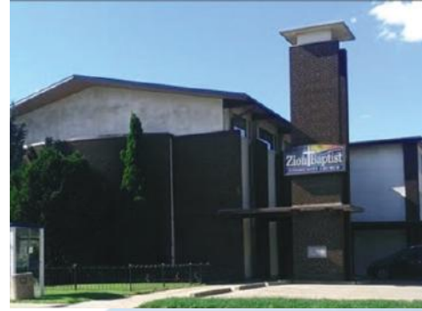
Zion Baptist Church 9802 76 Ave NW, Edmonton, AB
