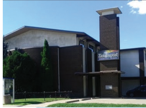
Zion Baptist Church 9802 76 Ave NW, Edmonton, AB
