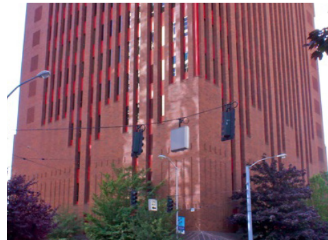
Building 2101 2101 2nd Avenue, Seattle, Washington, Belltown
