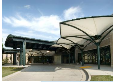
Muskogee Regional Medical Center 300 Rockerfeller Drive Muskogee, OK, USA 74401 Engineer: Lee & Browne Consulting Engineers Tulsa, OK
