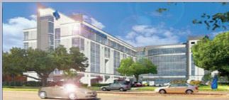
St-Joseph Women's Hospital Tampa, Florida www.sjbhealth.org Eng: Smith, Seckman, Reid Engineering
