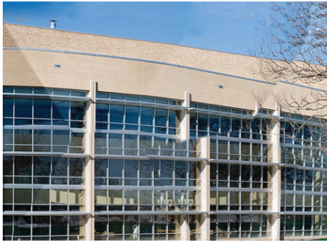
Research and Medical Clinic 4508 E. 41st Street Tulsa, OK, USA 74135 Engineer: Engineering Design Associates, Tulsa, OK
